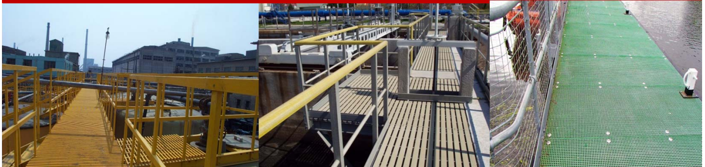
Oil / Gas / Chemical / Water / Wastewater Treatment Plants
